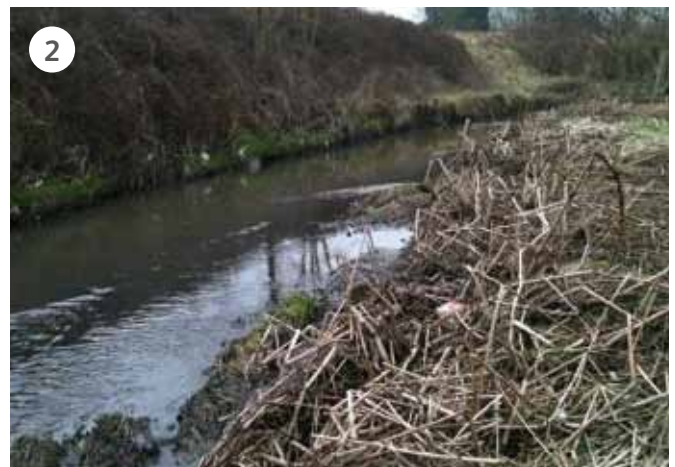
(1) Banks prior to removal of sheet piling; (2) The same banks post-removal
